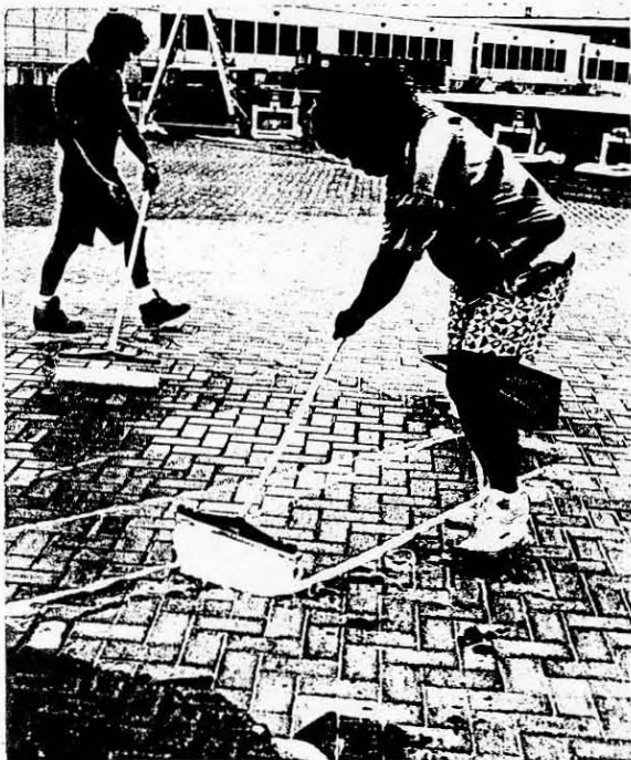
Figure 10. Applying urethane sealer.
