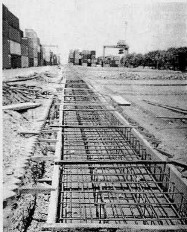
A new Transtainer track was being constructed
