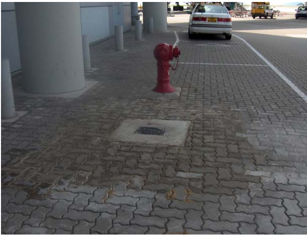
Figure 7. Maintenance at Service Pits (HKIA)
