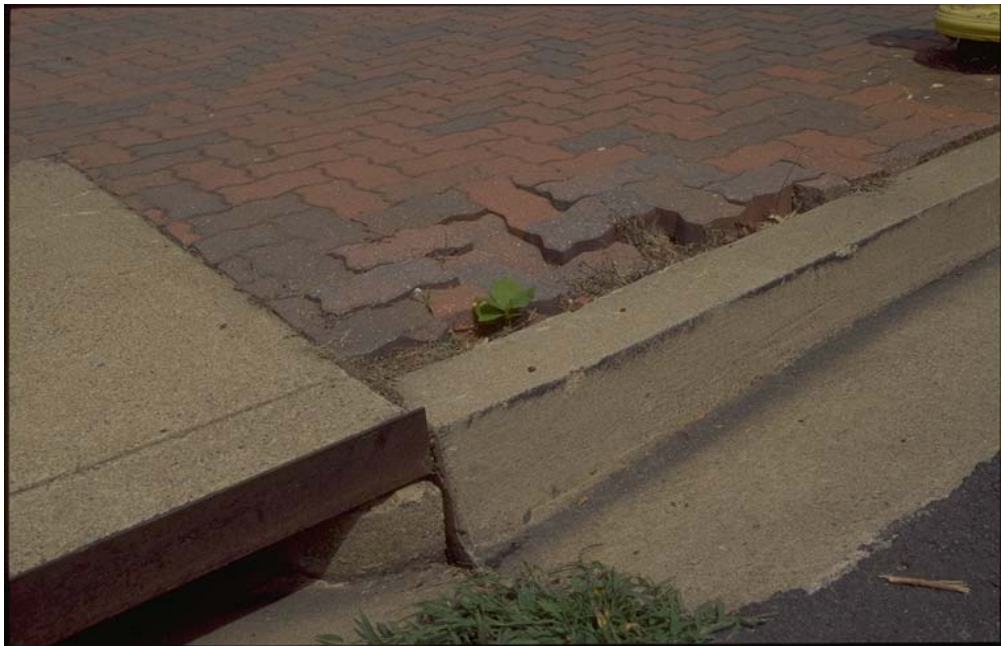
Figure 11: To prevent loss of bedding sand at the edge of curb, geotextile is recommended Source: Interlocking Concrete Pavement Institute
