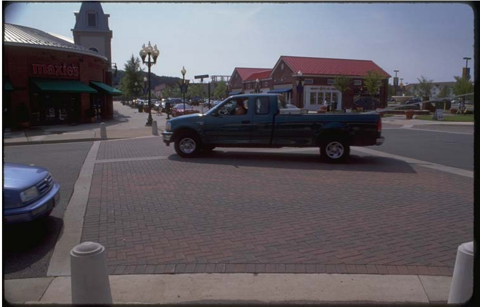
Figure 16: Concrete headers may be required at the edges of the cross walk depending on the amount of truck and bus traffic that is anticipated Source: Interlocking Concrete Pavement Institute
