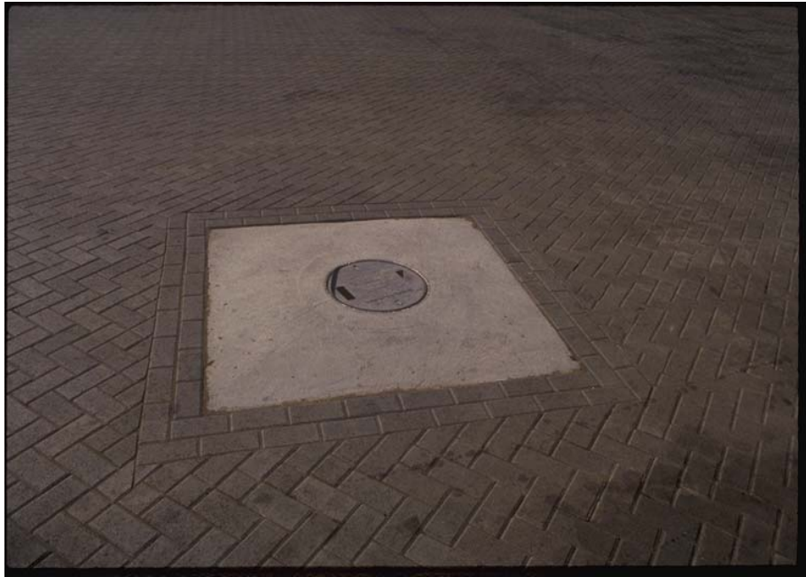
Figure 14: A concrete collar around a utility cover creates a better visual as well as eliminating settlement and cracking
