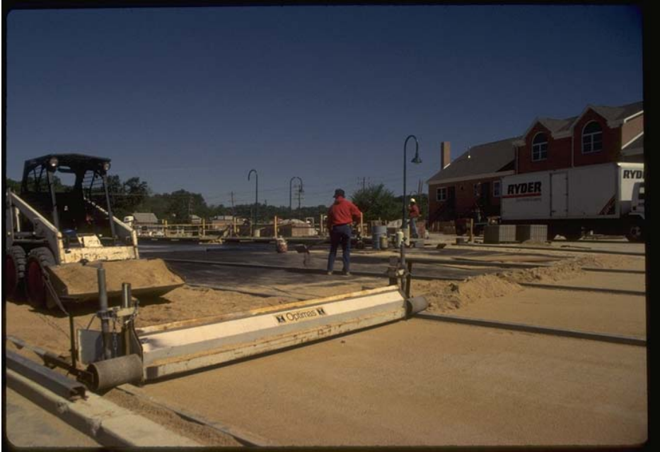
Figure 4: Mechanical screeding of bedding sand Source: Interlocking Concrete Pavement Institute
