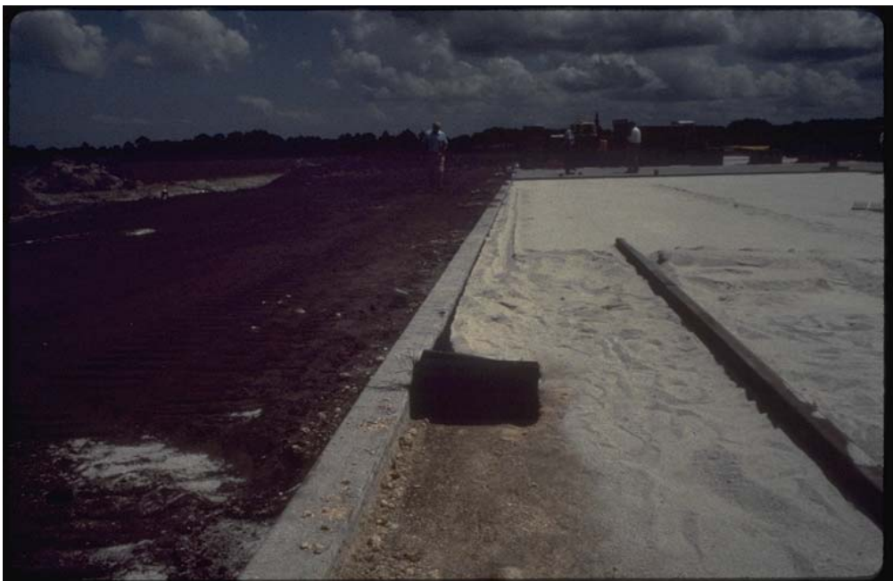
Figure 13: Geotextile shown at the interface of the curb to prevent loss of the bedding sand Source: Interlocking Concrete Pavement Institute
