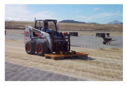
Figure 9. Spreading joint sand with mounted brooms.
