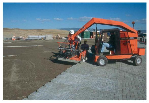
Figure 4. Mechanized equipment placing interlocking concrete pavement.
