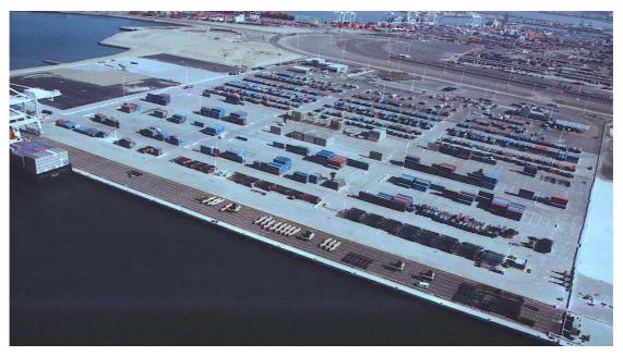
Figure 2. The first phases of the paving at Berths 55/56 consisted of 170,000 m<sup>2</sup> of concrete pavers.
