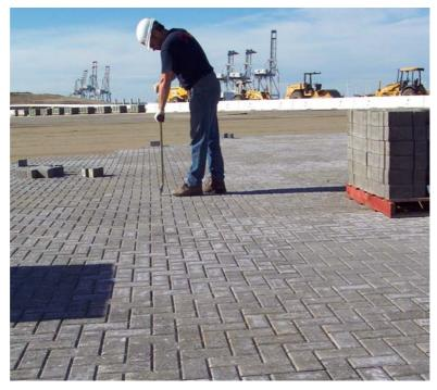
Figure 6. Straightening joint lines prior to initial compaction.
